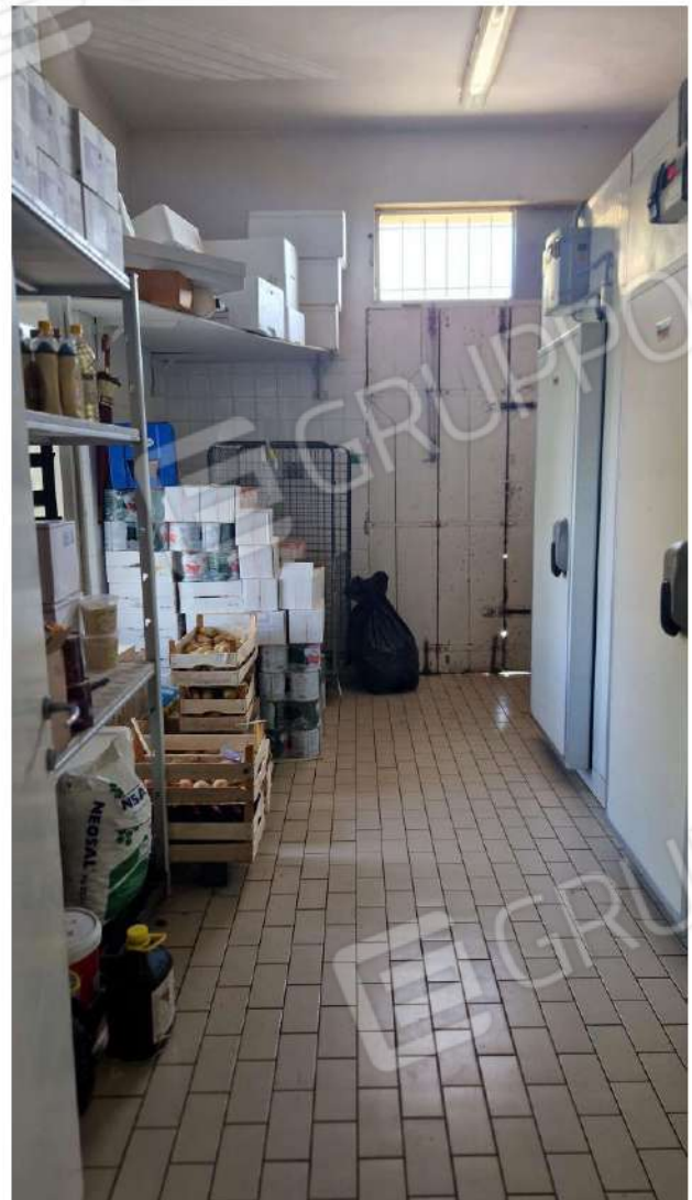
Locale celle frigo
