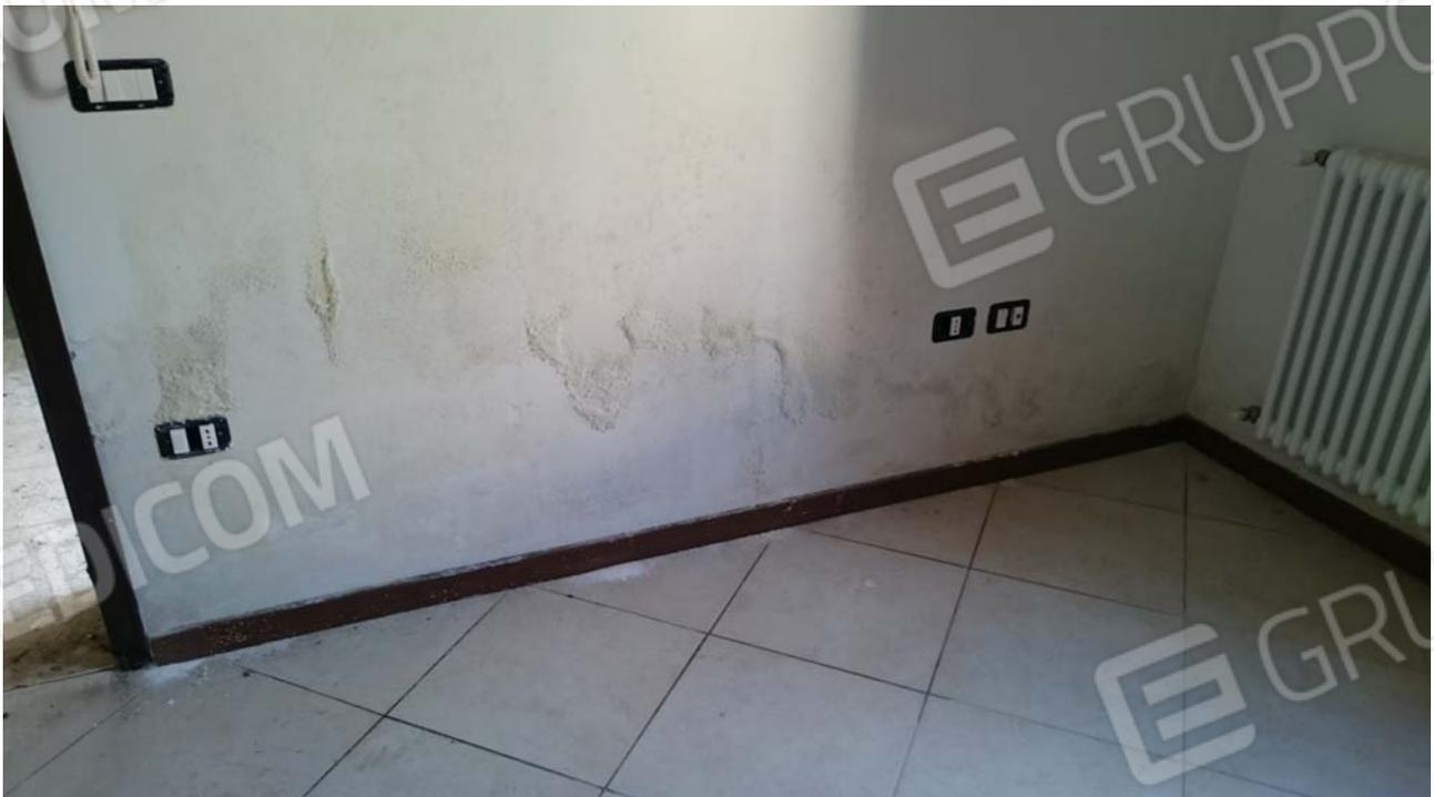
ALLOGGIO SUB 30 P.1° PRESENZA DI UMIDITA'
