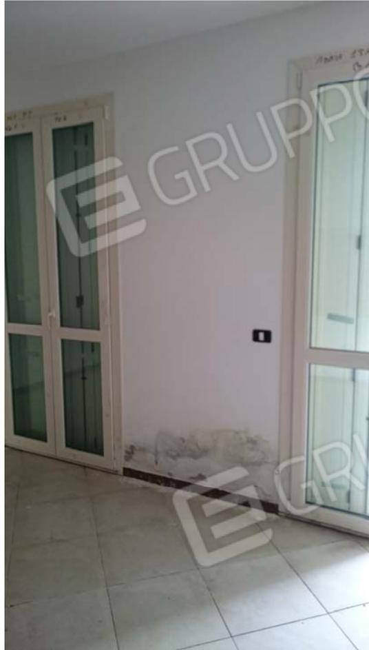
ALLOGGIO SUB 36 P.1° PRESENZA DI UMIDITA'
