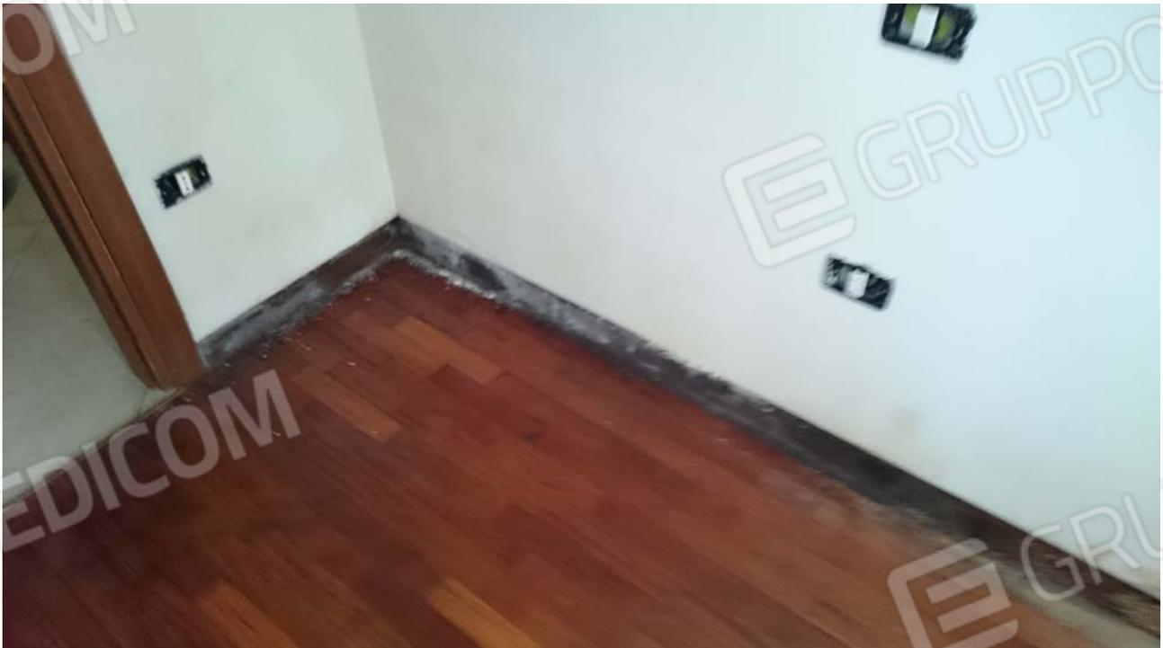
ALLOGGIO SUB 26 P.T. (PRESENZA DI MUFFE)
