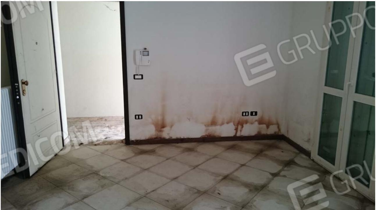
ALLOGGIO SUB 27 P.1° (PRESENZA DI UMIDITA')
