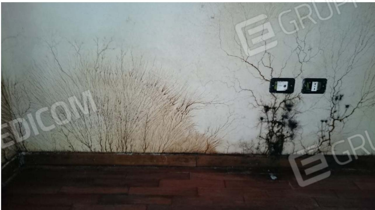
ALLOGGIO SUB 23 (PRESENZA DI MUFFE)
