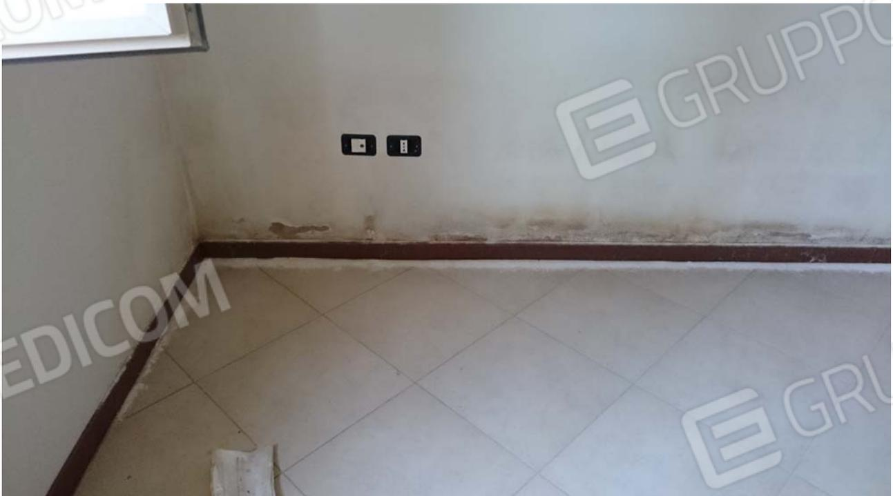
ALLOGGIO SUB 33 – PRESENZA DI UMIDITA'
