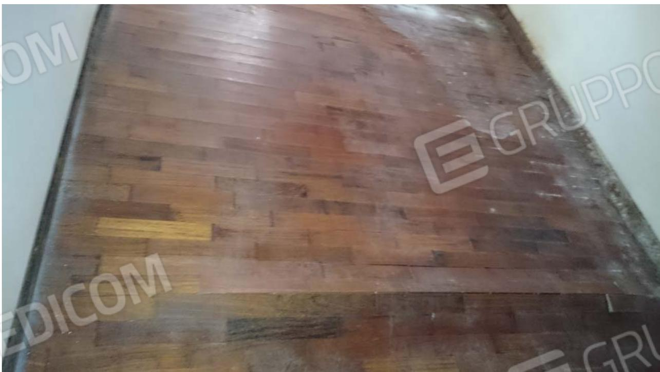
ALLOGGIO SUB 24 (PRESENZA DI UMIDITA' DI RISALITA)
