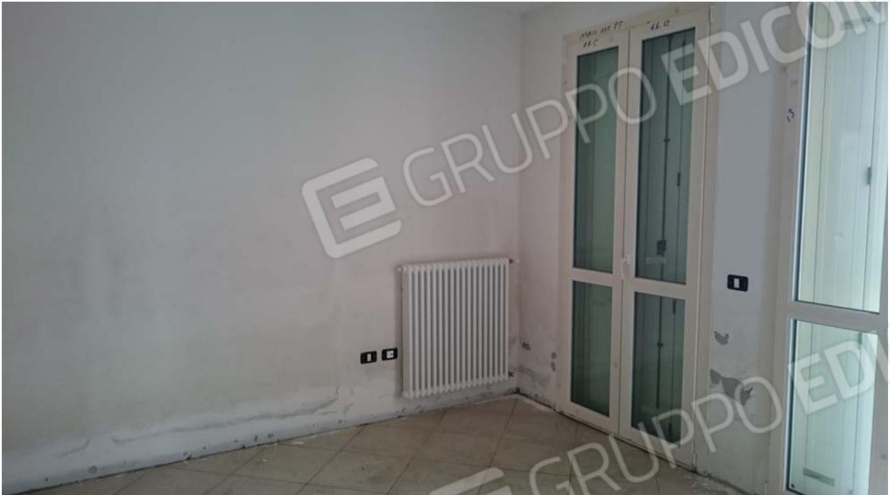
ALLOGGIO SUB 32 – P.1° PRESENZA DI UMIDITA'
