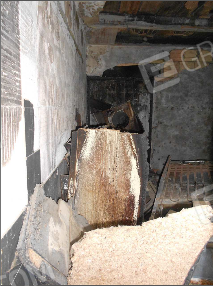
Locale a piano terra
