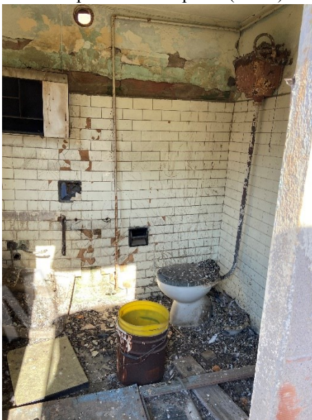
Sub. 13 – locale wc P1
