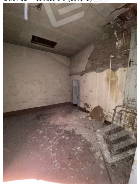
Sub. 13 – locale P1 (foto 3)
