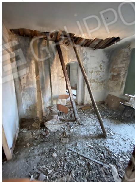
Sub. 13 – locale P1 (foto 1)
